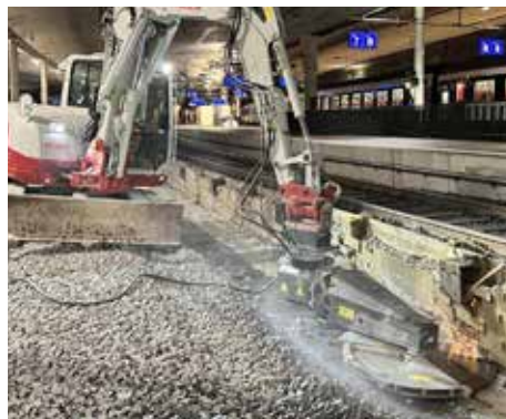
The CMS diamond tool saw arm easily cuts vertically, horizontally, and diagonally.
