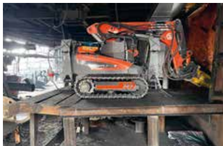
Safe entry of the machine in the kiln.
