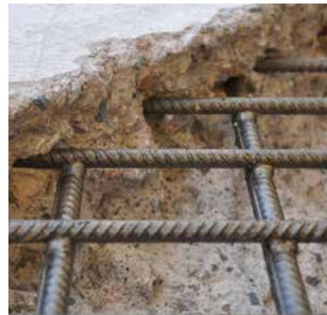
Hydrodemolition robots can be programmed to remove only unsound concrete, which minimizes waste.
