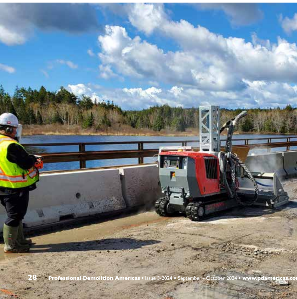
Hydrodemolition robots can be programmed to remove only unsound concrete, which minimizes waste.
