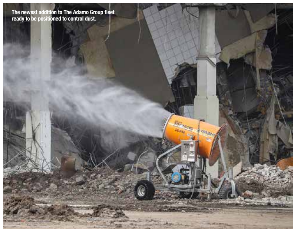
The vertical angle can be adjusted to cover activities on the ground or at the rooftop.
