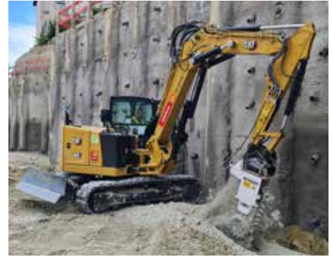
Image to the right: Along the foot of the bored pile wall, a drainage trench is excavated – saving time and money with a 9-t excavator and KEMROC EK 40 chain cutter.
