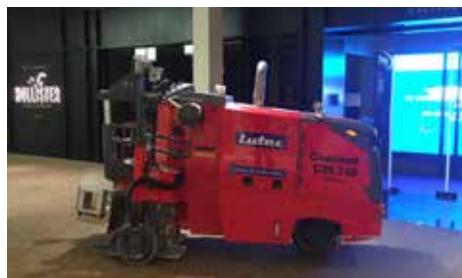
Removing concrete in the second floor with the CM 140.
