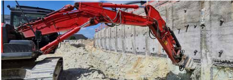
Layer by layer, the areas of quartzite rock between the bored piles are exposed. After lining with steel mesh, shotcrete is applied. The amount of shotcrete used is kept to a minimum.
