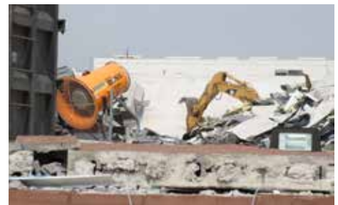
The vertical angle can be adjusted to cover activities on the ground or at the rooftop.
