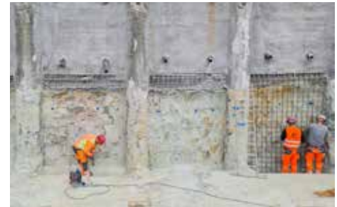
Layer by layer, the areas of quartzite rock between the bored piles are exposed. After lining with steel mesh, shotcrete is applied. The amount of shotcrete used is kept to a minimum.
