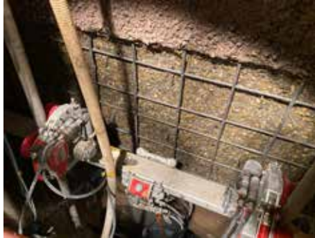
Restocrete's Nick and Justin Downar needed an efficient hydrodemolition machine that could be operated from a safe distance above the chamber, so they turned to the Aquajet Ergo. Photo credit: Restocrete, Inc.
