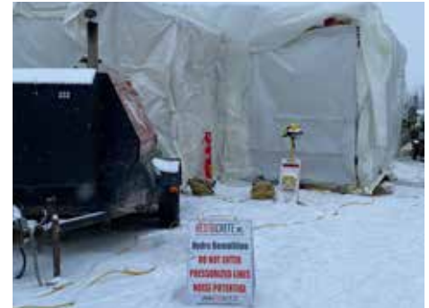
The Restocrete crew constructed an insulated shed for the Ergo and Jetstream pump, with heaters running throughout the project to combat extremely cold temperatures. Photo credit: Restocrete, Inc.
