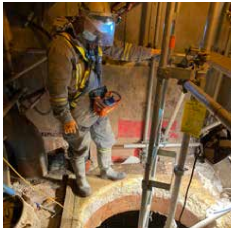
Thanks to the Ergo's remote-control capabilities, the Restocrete crew could operate the equipment safely from above, reducing time required in the pit. Photo credit: Restocrete, Inc.
