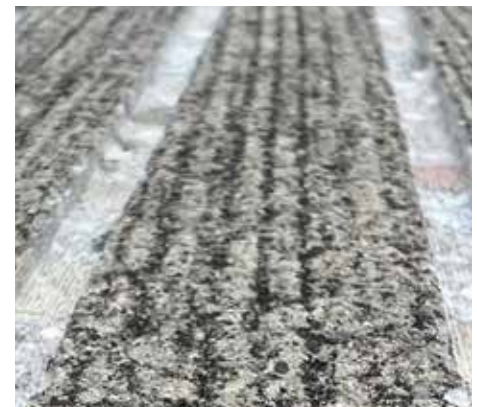
The final grooves for improved drainage.
