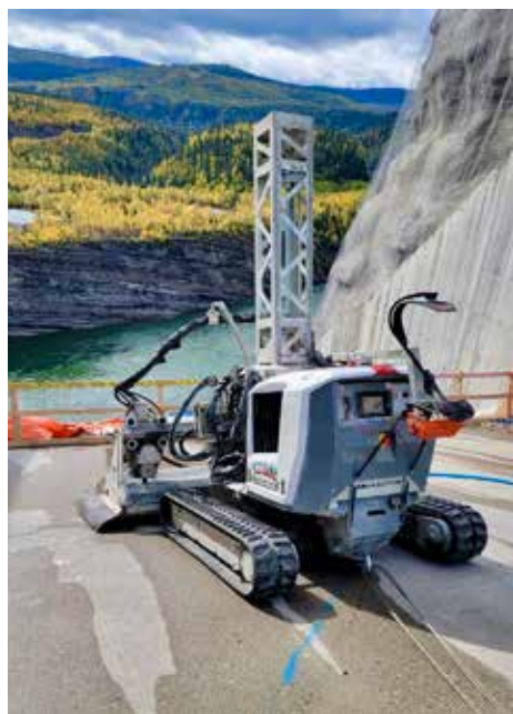
The hydrodemolition robot set up for the 2021 try-out on a 9.8-ft (3m) spillway crack
