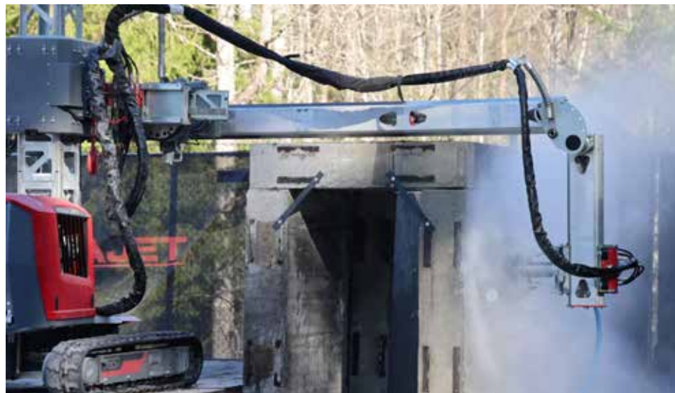
Below: The Extension Kit can be configured several ways with an elbow and beams, allowing the operator to perform hydrodemolition in hard-to-reach areas.
