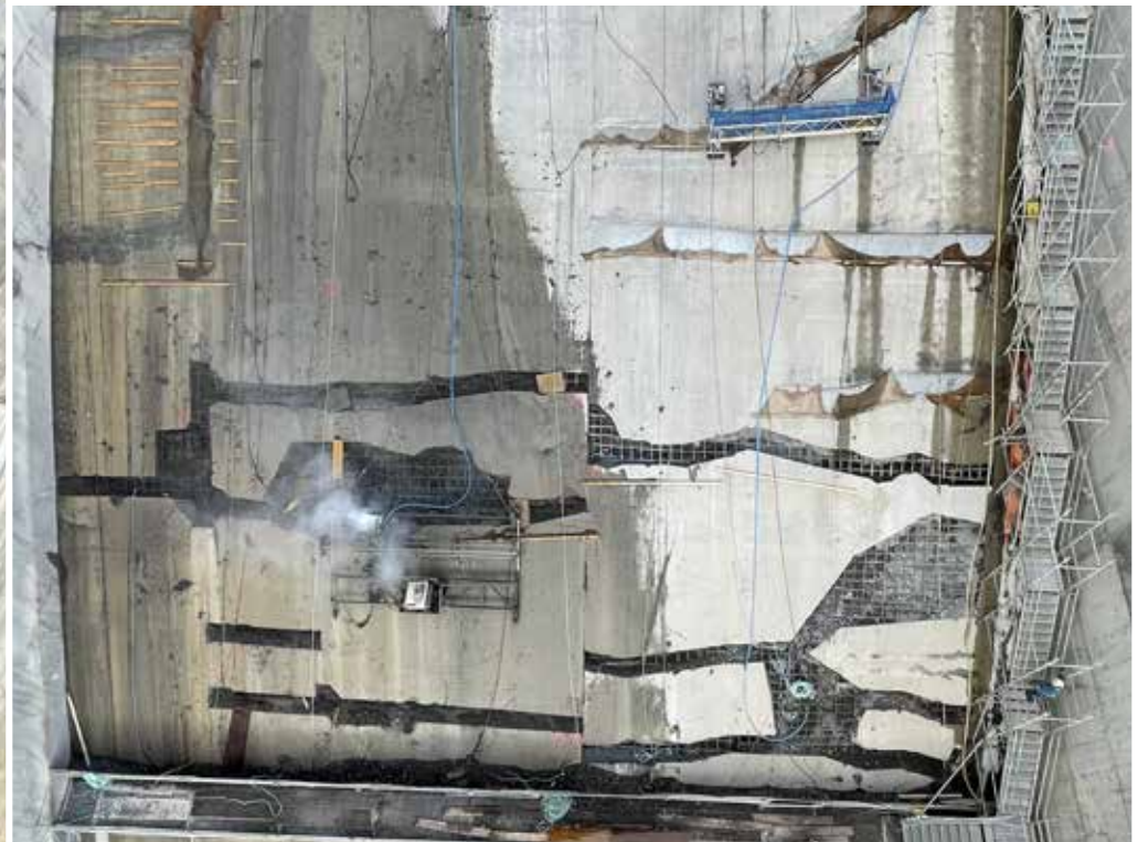
Crack repair work on the slope of the spillway at the W.A.C. Bennett Dam.
