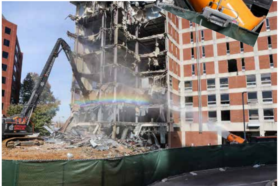
The DB-60 Fusion effectively suppressed dust particles during the demolition.
