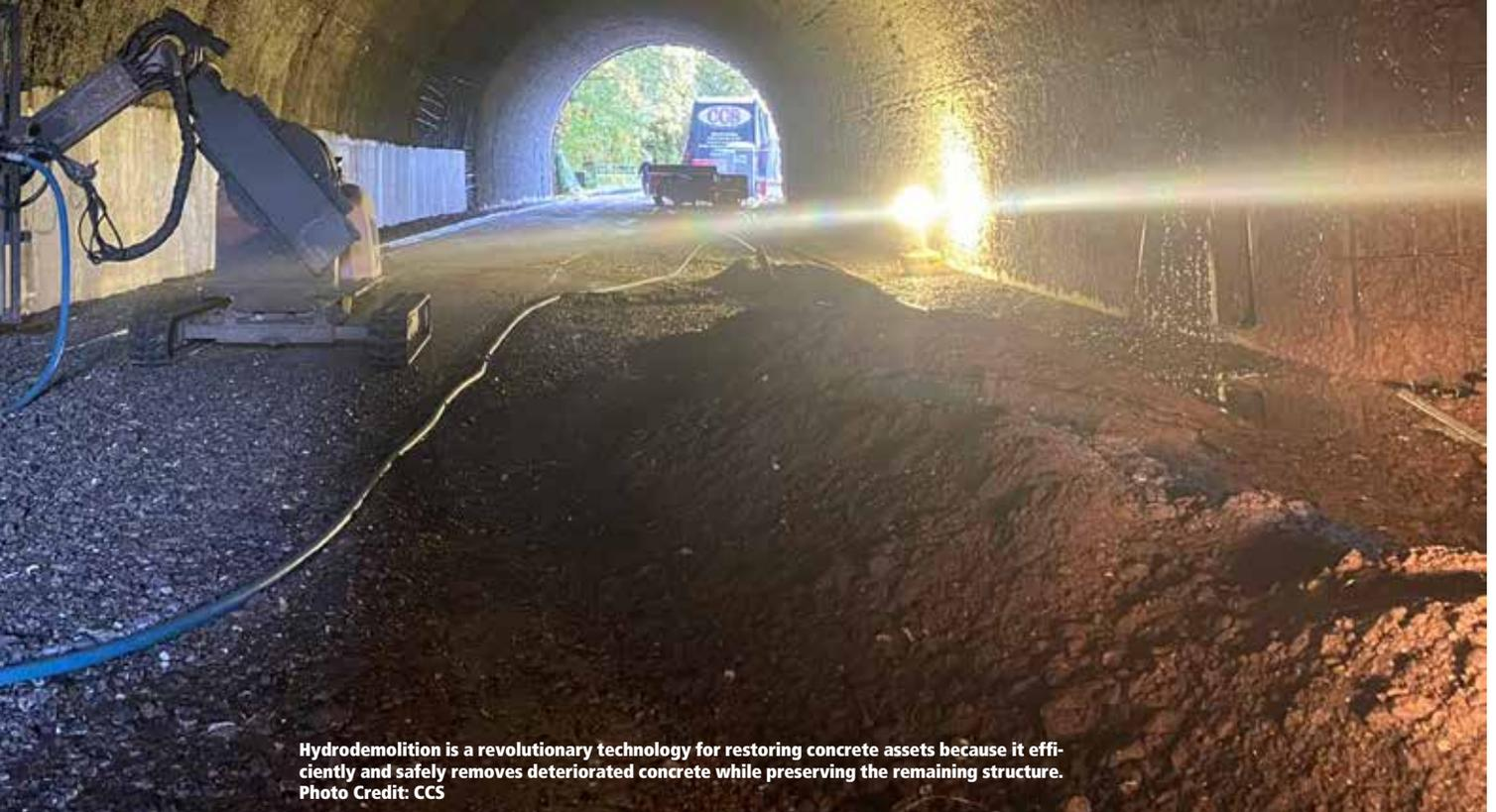
**Hydrodemolition is a revolutionary technology for restoring concrete assets because it efficiently and safely removes deteriorated concrete while preserving the remaining structure.**
