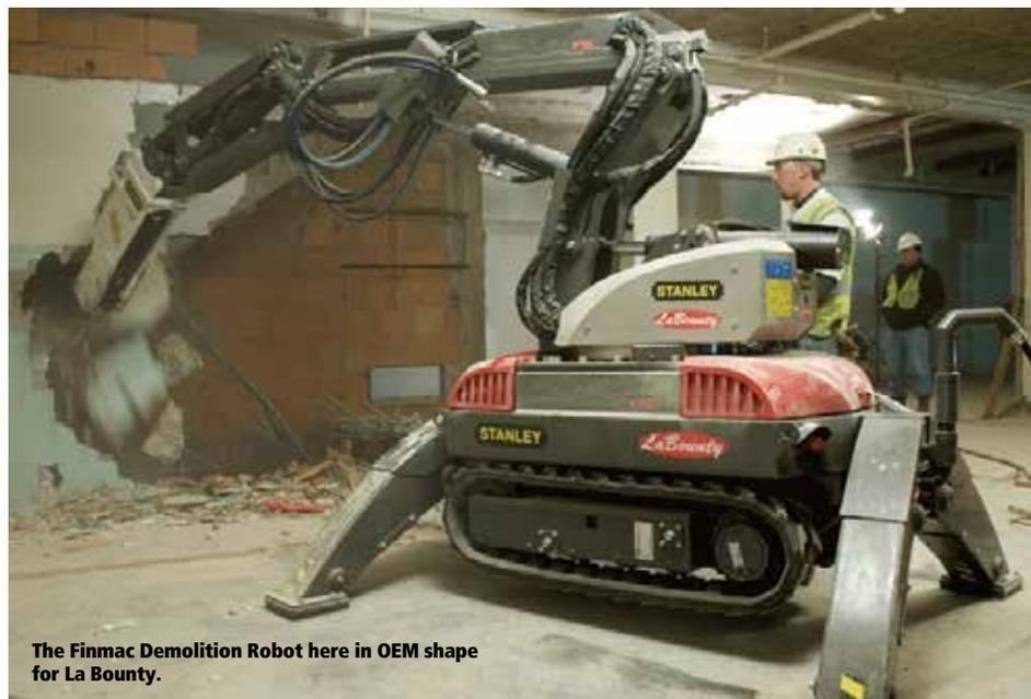
**The Finmac Demolition Robot here in OEM shape for La Bounty.**
