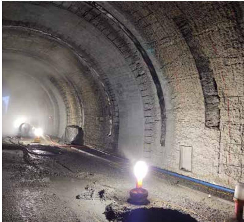
**Tunnel 2 restoration work was performed in phases to create new structural bracing, while also maintaining the Tunnel's integrity during construction. Photo Credit: MJ Hughes Construction**
