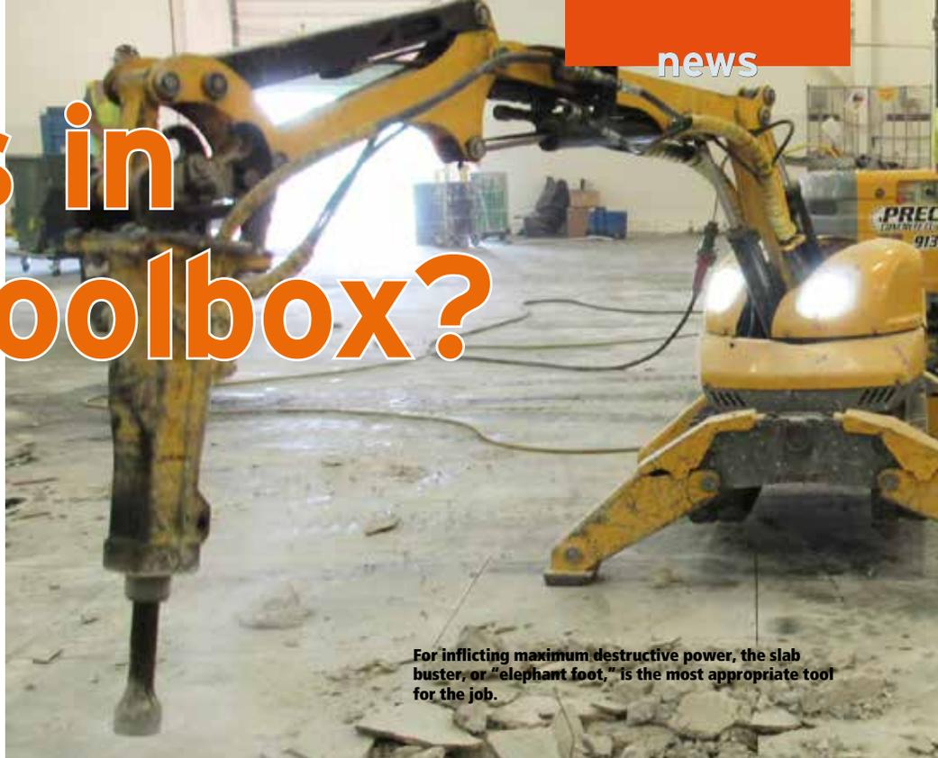
**For inflicting maximum destructive power, the slab buster, or "elephant foot," is the most appropriate tool for the job.**
