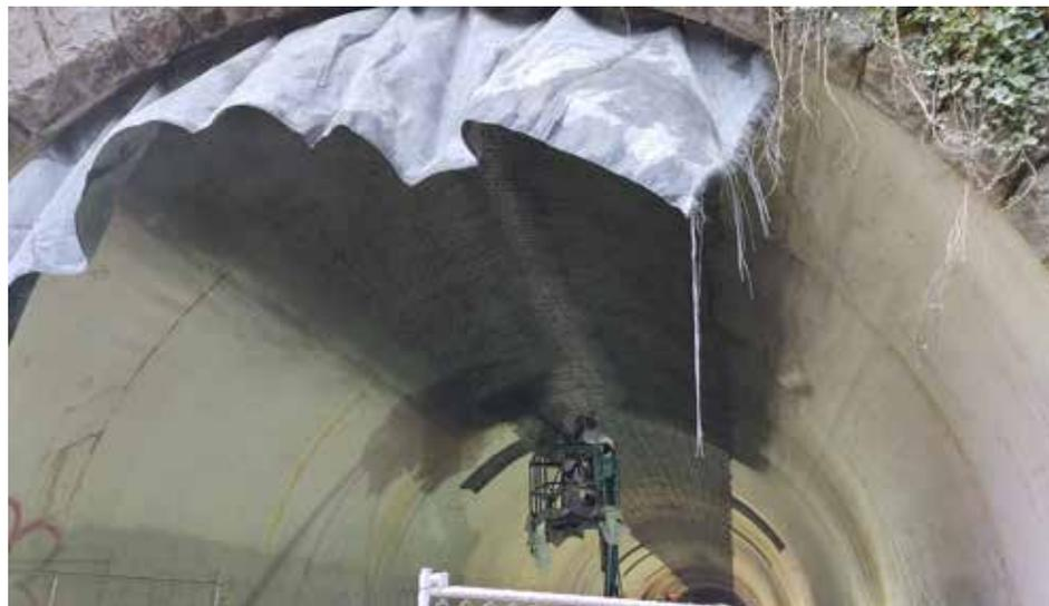
**A new layer of Shotcrete was installed which will seal up the rebar and protect it against penetration of harmful contaminants for many years to come. Shotcrete, also known as gunite or sprayed concrete, is concrete or mortar conveyed through a hose and projected at high velocity onto a surface. Photo Credit: MJ Hughes Construction**
