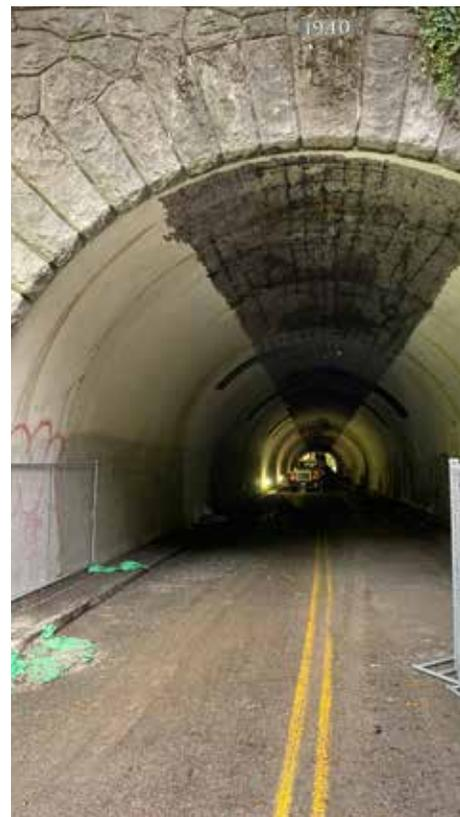
**The Tunnel 1 renovation plan called for a 14 ft wide x 2 in deep strip to be removed at its curved crown for the entire length of 500 feet. Photo Credit: CCS**
