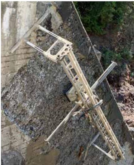
**Contractors can use an Aqua Spine for concrete removal in areas that are inaccessible to Hydrodemolition robots. This multi-modular system features a single feed beam to ensure adaptability to different applications. Photo courtesy of Beartooth Water Jetting and Video Inspection.**
