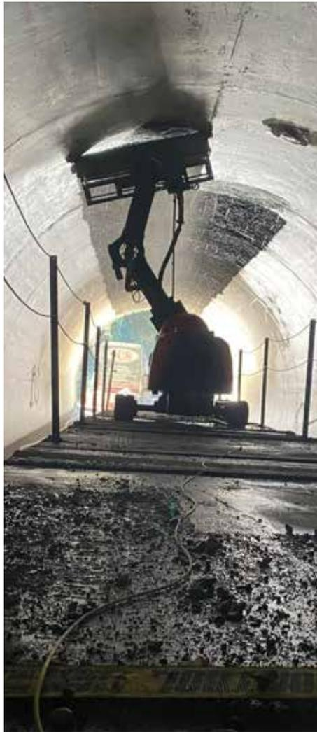
**The versatility of the Conjet 557 MPA was important, as CCS utilized the Multipurpose Arm for reaching different angles and distances, the extendable tracks for stability, and multiple speed zones traversing the cutting head to ensure an even removal along the curved tunnel radius. Photo Credit: CCS**
