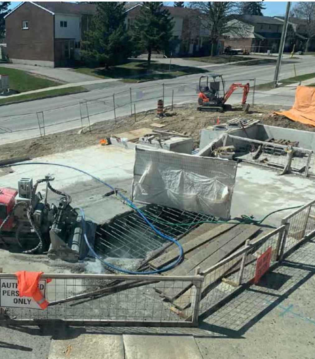
Hydrodemolition saves Drewlo about 40% of the time compared to using a scarifier or other mechanical means, allowing the team to move on to subsequent tasks that much faster.
