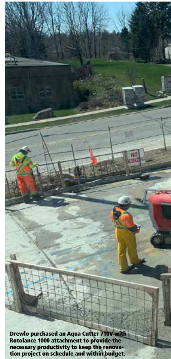
Hydrodemolition cleans and descales rebar without damaging it or causing microfractures, saving Drewlo an estimated $40,000 per structure.
