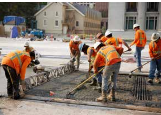
New concrete is applied over the hydrodemolition area, strengthening the parking deck roof and preserving the structure for many years of continued use. Photos: Intellectual Reserve, Inc.
