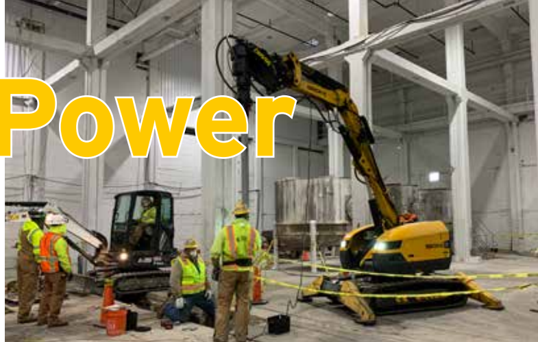
The Brokk 500's 23-foot (7-meter) reach allowed Drilling Service Co. to access helical pier locations that would have been challenging with traditional mono-boom equipment. This included reaching up, over or around existing equipment in the building when necessary.
