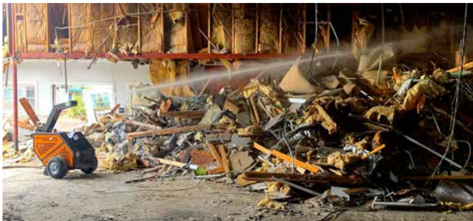
The DustBoss Atom ™ controls dust on storage piles during the separation process for recycling.
