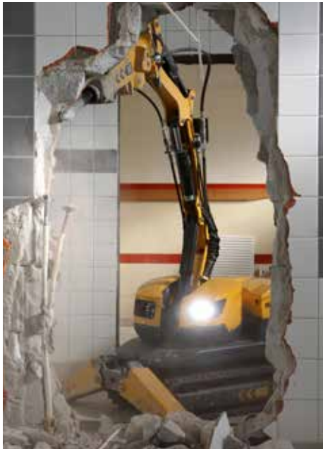
Thanks to advanced technology and an industry-leading power to weight ratio, compact demolition robots can access some of the most restrictive jobsites — including those with dust, vibration and noise restrictions as well as low floor loads.
