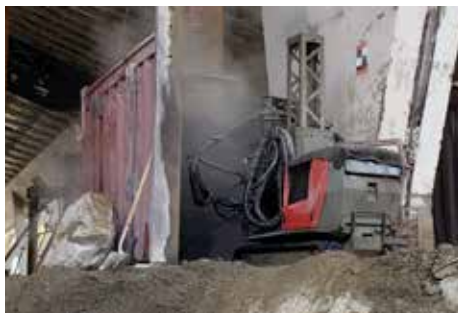
For precision and efficiency, the contractor used two AquaJet Aqua Cutter 710V robots to remove portions of 28 columns, four chevrons and one buttress in 30 days.
