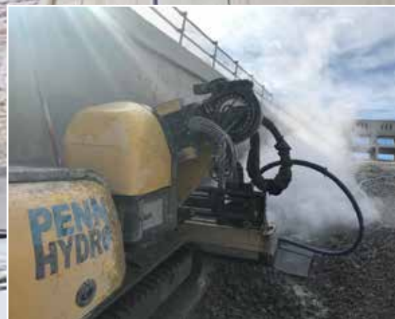
Robot 557 removes concrete from the spillway.
