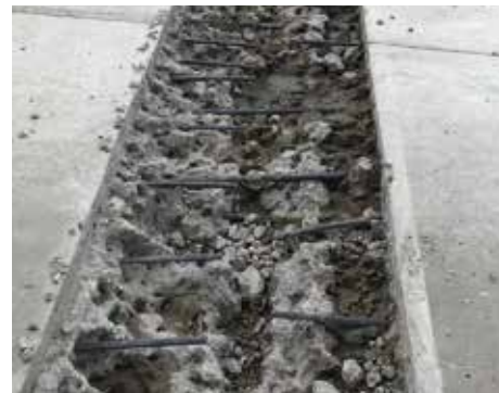
Structural joint opened using hydrodemolition.
