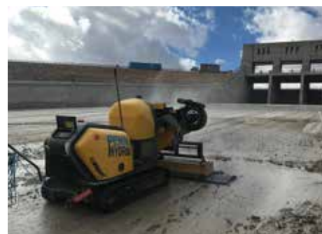
Robot 557 and the Hammelmann Power pack on the dam crest.
