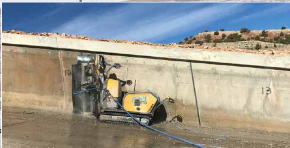
Conjet equipment on the job at the Alcova Dam project in Wyoming (see p. 25) A Robot 557 removes concrete from the wall in minutes.
