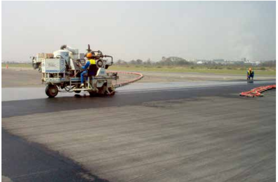
Runway grooving on a US military base on the island of Diego Garcia, in the middle of the Indian Ocean.
