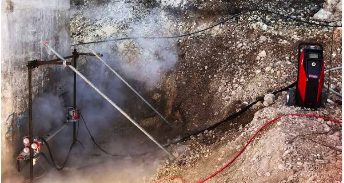
With robotic water blasting, the heavy lifting is left to the machines while crew members stand safely out of the way.
