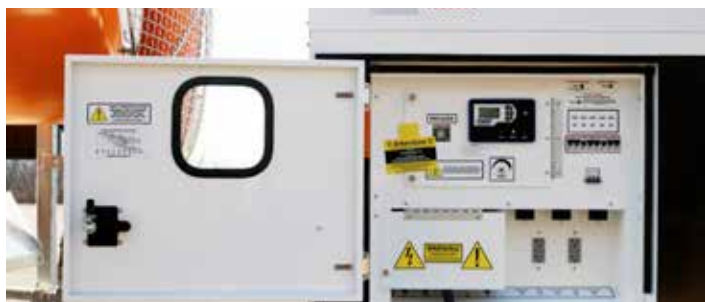
The touch-screen control panel is protected in a NEMA 3R cabinet
