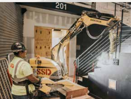
SSD used an Atlas Copco SB 202 hydraulic breaker attachment, and the unique Brokk three-part arm design allowed them to take advantage of extended reach capabilities and precise demolition. Photo courtesy of Brokk.
