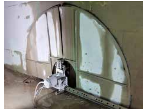
London Diamond Drilling used tracksaws for the perimeter of the site.
