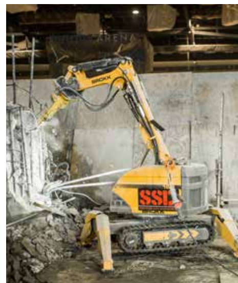
Above: SSD knew using remote-controlled demolition machines would improve productivity over handheld tools, as well as keep workers safe from flying concrete and fall risks. Photo courtesy of Brokk.
