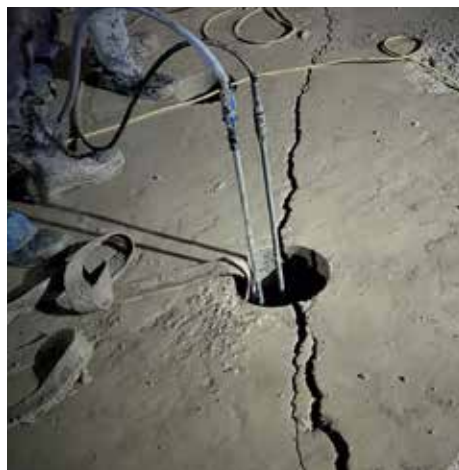
Dymatec's 8" hydraulic burster successfully breaking up a thick slab of concrete.
