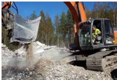
Tatu Kantola crushes concrete with Viper VPCH 21.
