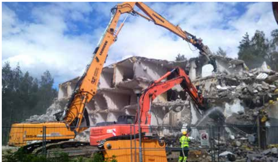
First phase was to tear down the building to blocks approximately 31.5-in (800 mm) in size. Water suppression was mandatory due nearby population and housing
