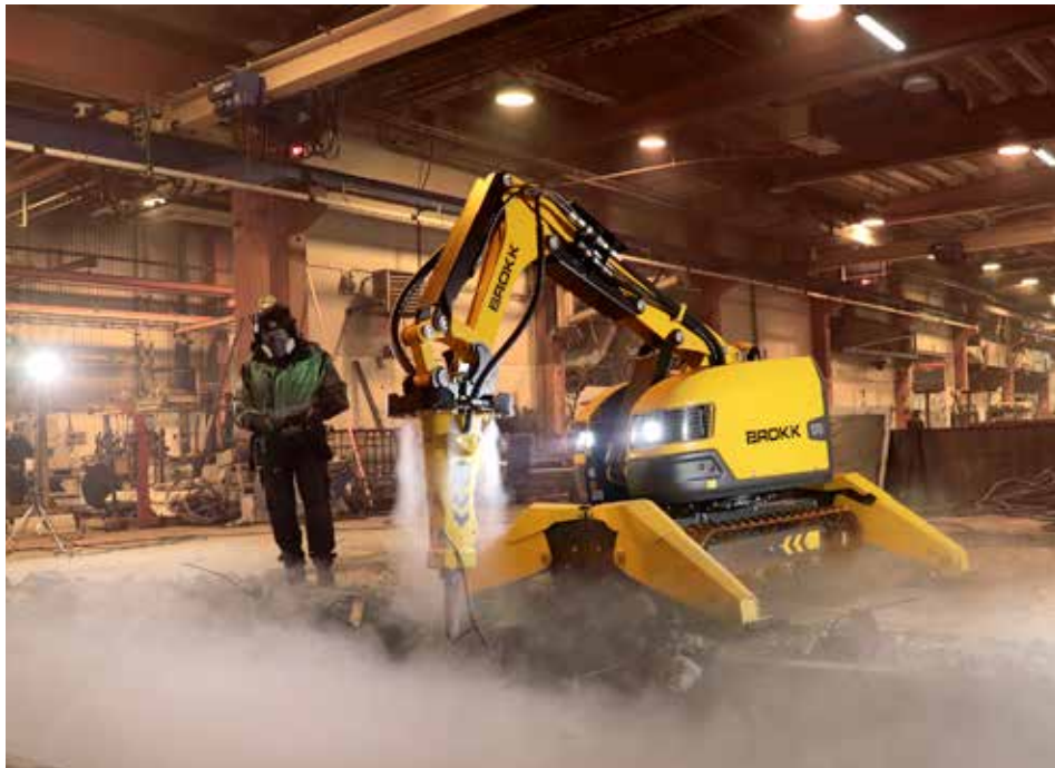
Brokk Atomized Water Mist System produces atomized fog that effectively binds airborne dust particles while also providing ground-level dust suppression. Additionally, the mist dissipates, rather than forming puddles, for a safer, cleaner jobsite.
