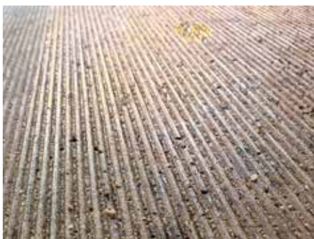
Clean cut edges and an optimal grinding pattern.
