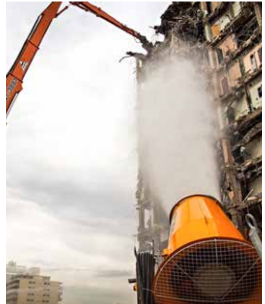
An excavator with a hydraulic demolition attachment quickly takes the building apart.
