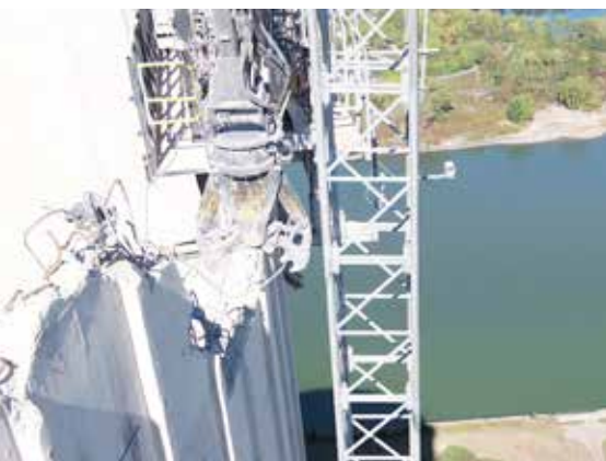
Working with the 1t Konverma HCM 600-M shear.
