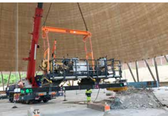
It took about 14 hours to lift the robot and equipment to the top of the chimney.
