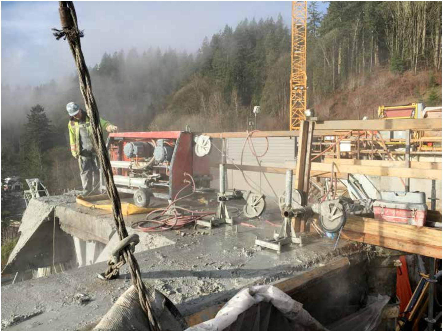
Concrete sawing and drilling work involved the cutting and removal of four existing piers, the bridge deck and sections of the spillway.
