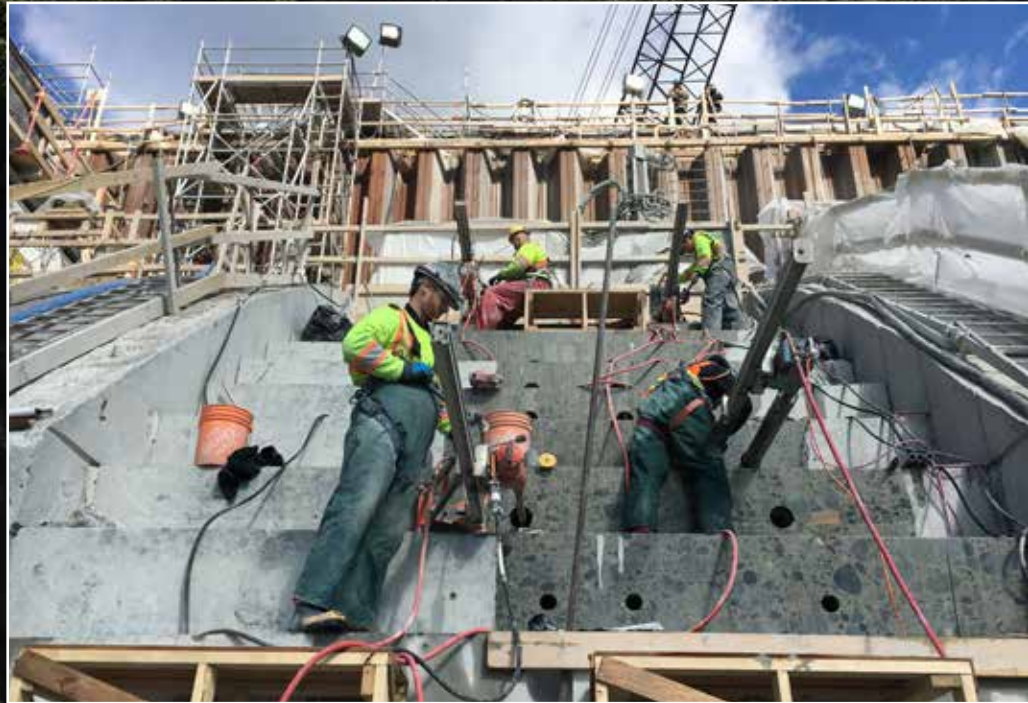
New steps were cut in the 60-degree sloped dam wall for the installation of new steel formwork.
