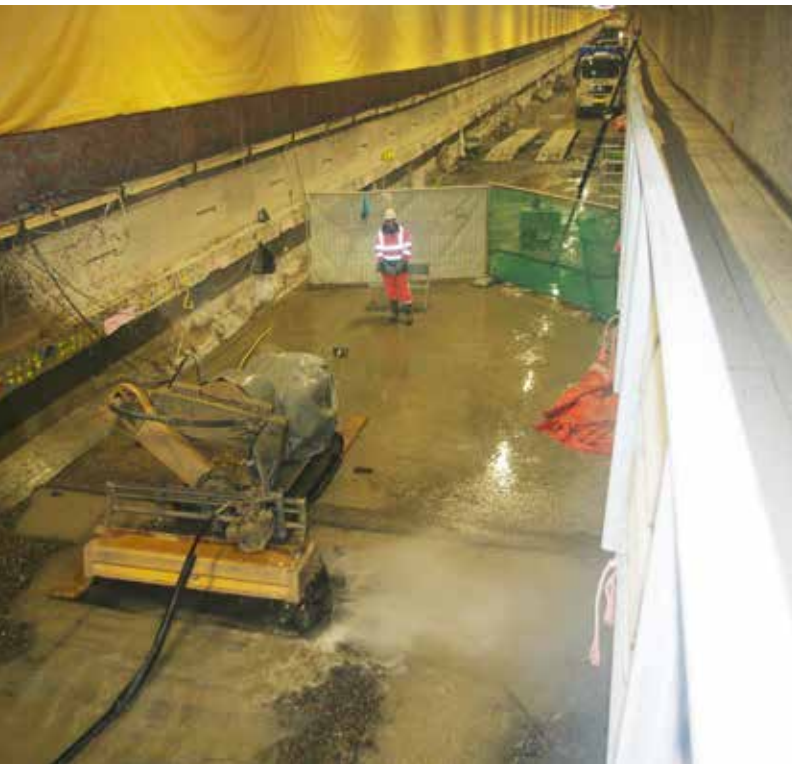
The Conjet Robot 557 is being used to remove the top layer of the concrete floor in the underwater tunnel.
