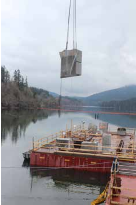
Cut sections were removed by crane and placed on a nearby floating barge.
