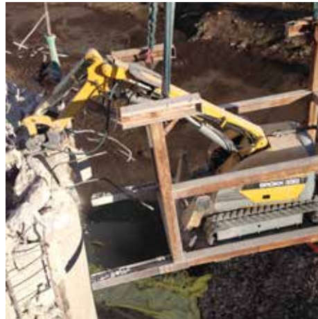
A contractor attaches the Brokk 330D demolition robot to a custom platform and lifts it with a crane, using the breaker attached to the machine's three-part arm to chip away at the concrete silo.
