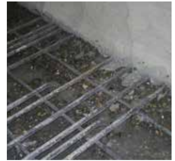
Hydrodemolition has been chosen as the most viable and efficient demolition method because of less noise and dust, and to avoid cracks in the tunnel structure whilst maintaining the original rebar.
