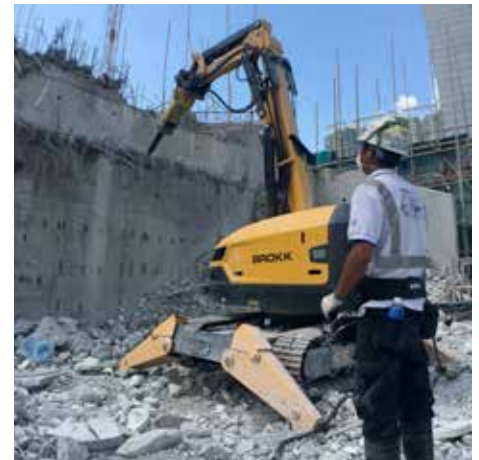
Contractors can operate the Brokk demolition robot's three-part arm with attachments for breaking, cutting and a number of other applications from a safe distance.
