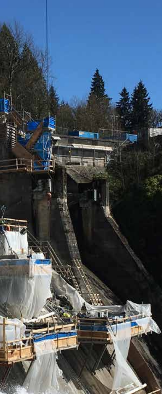
New steps were cut in the 60-degree sloped dam wall for the installation of new steel formwork.
