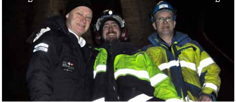
Lars-Göran (left), together with some clients, in his right environment renovation turbines in a Swedish power plant using hydrodemolition techniques.
