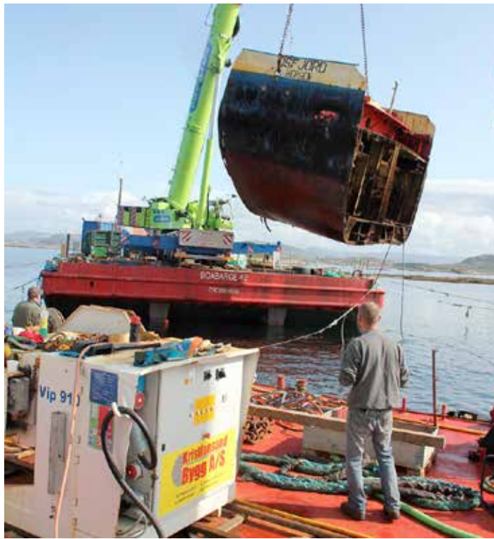
The shipwreck was cut into several parts in order to bring it ashore safely.
