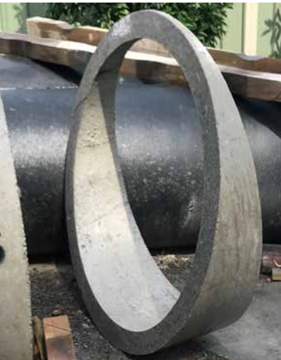
A 15° pipe cut.
