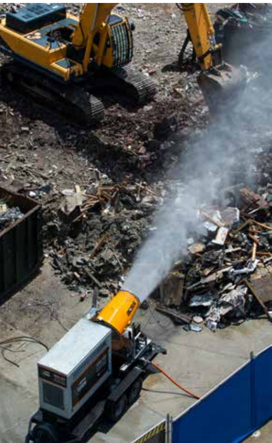
Atomized mist effectively suppresses fugitive dust in the air and on the ground, without excessive runoff.
