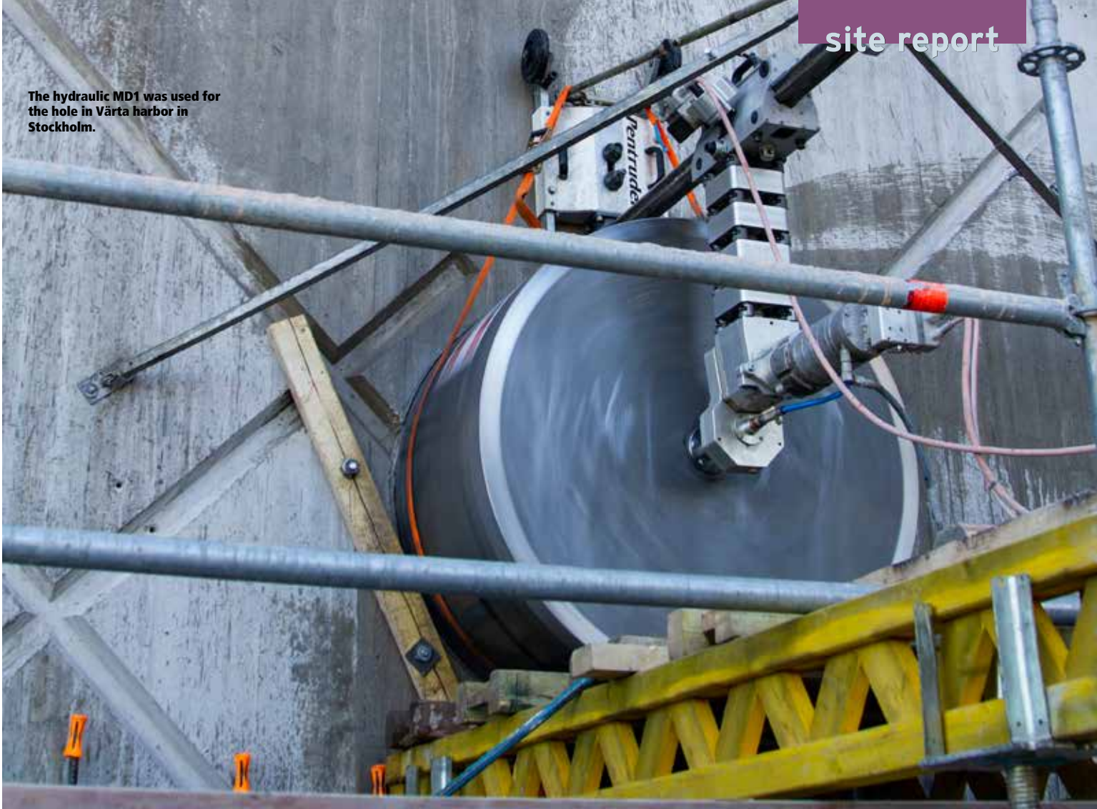
Above the Pentrunder MD1 heavy duty core drill, a 15 kW HF motor and auto feed, the 47-in (1,200 mm) diameter cutter took less than 2h to complete.
