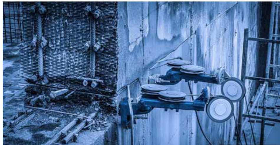
Dismantling of 22 running meters of reinforced concrete walls. (Photo: Diamond Drilling).
