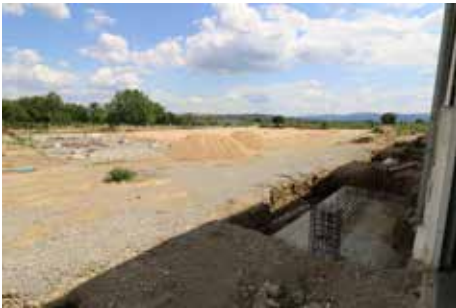
New land ready for construction in Krun.
