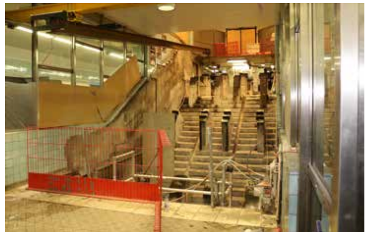
Every older escalator to be replaced has an average of 12 concrete foundations to be wasted. Each foundation weighs between one to two tons.
