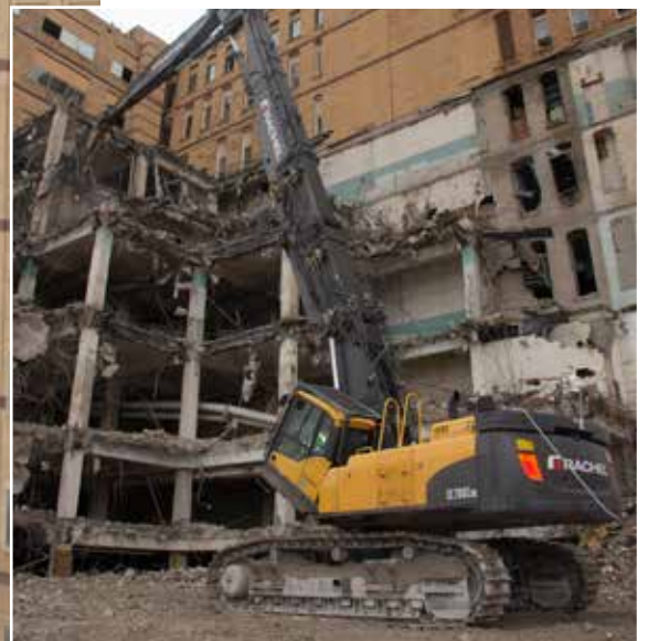
The high-reach excavator takes down the concrete beams with ease.
