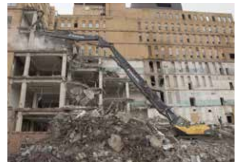
The EC700CHR excavator uses 464-hp (346kW) of power, plus perfectly harmonized hydraulics to make light of the heavy-duty task.
