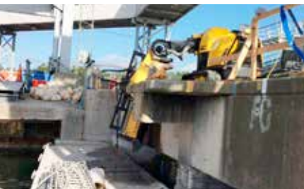
The Conjet Robot is positioned and ready to execute the removal down to 1.2 in (30mm).
