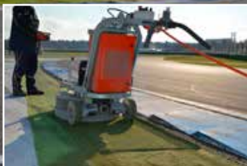
Thick lacquer layers needed to be removed around the circuit.
