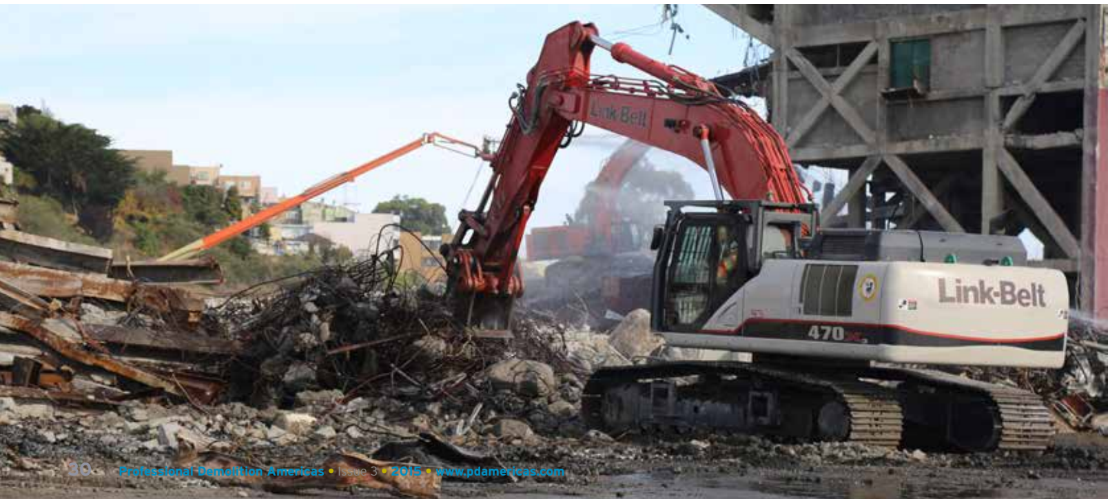
Below: An Link Belt excavator sorts rubble from Candlestick Park before it's crushed onsite or shipped out for additional processing—roughly 98 percent of the material will be reused or recycled.
