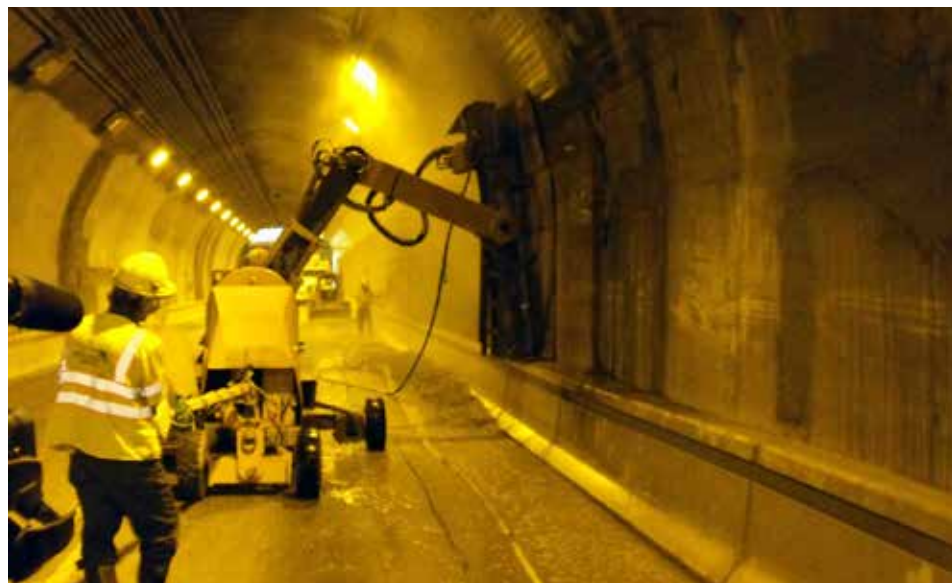
Two Conjet Robot 363 hydrodemolition machines have been adapted to suit the curvature of the horseshoe-shaped walls of the two Liberty Tunnels.
