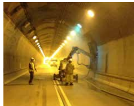
Two Conjet Robot 363 hydrodemolition machines have been adapted to suit the curvature of the horseshoe-shaped walls of the two Liberty Tunnels.
