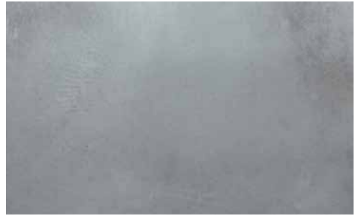
Close-up of an industrial floor finish.
