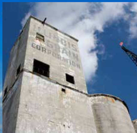
The three silos and one grain elevator sat within five feet (1.5m) away of several combustible fuel tanks.
