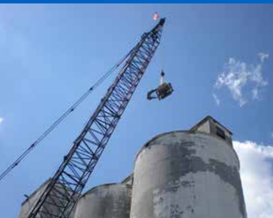
The Brokk 180 was hoisted by a crane to the top of the silo to begin demolition of the roof.
