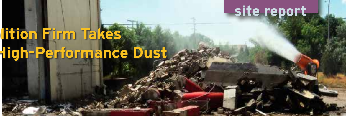
Veit reports far better dust control than with manual spraying, as well as significant labor savings.
