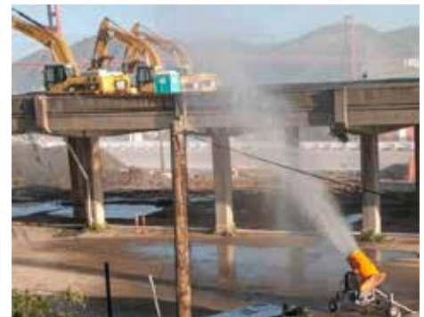
When completed, the new parkway will reveal striking views of the Presidio and San Francisco Bay.
