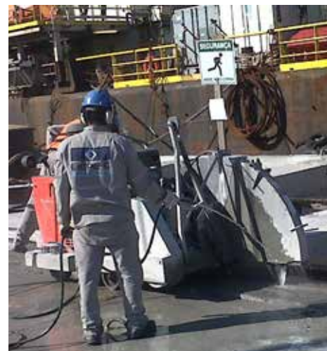
Cutting with FS 9900 was quite efficient — as much 66ft (20m) per hour.
