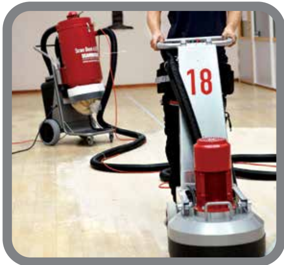
Grinding wooden floors and parquet flooring with Scanmaskin 18
