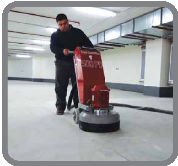
Removal work and floor preparation with Scan Combiflex 500PD
