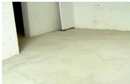
Photos of the apartment after leveling with the Husqvarna PG280.
