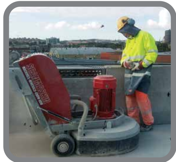
Grinding of bridges and car park areas with Scan Combiflex 1000RC
