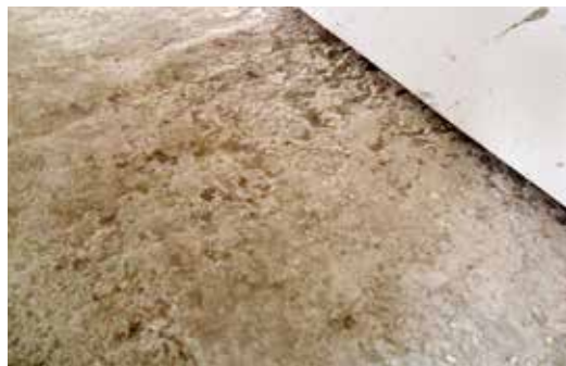
Floor apartment before grinding with the PG280.
