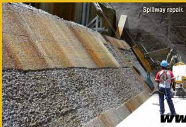
A Conjet Robot operated from a platform specially designed by the contractor, with advice from Conjet, to cater for the geometry and slope of a spillway channel at the Guri dam, which have an average slope of 51°.
